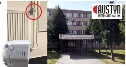
Temperature, humidity, and CO<sub>2</sub> sensors are installed in classrooms. When detecting worsened conditions, the system automatically exchanges air using a recuperation unit. Window opening sensors are installed on the windows to prevent unnecessary heating.
